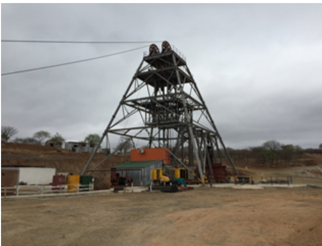
Exhibit 6: Temporary headframe at Central Shaft
