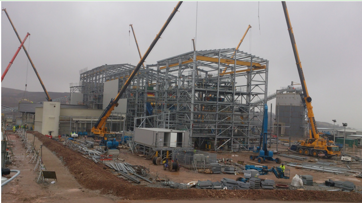
Exhibit 1: Hemerdon's processing plant is under construction
